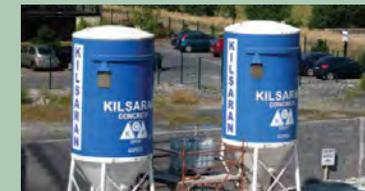
**05** Use of mortar silos to reduce water usage
