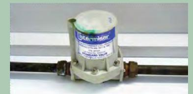
**09** Install an automatic urinal flushing device or use waterless urinals
